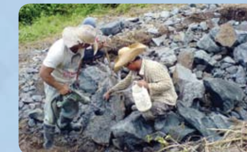
Stonewall building or tuping is a remarkable indigenous engineering skill among the Cordillera Igorots, who developed the expertise through centuries of building rice terraces and stabilizing steep mountain slopes. It involves laying a strong foundation, called pegnad , that is crucial in ensuring the stability of the stonewall, then piling and fitting stones together in a neat and systematic way. The tuping is integral to the sustainability of indigenous livelihoods and communities in the Cordillera.
